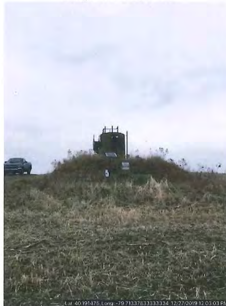
Photo #12 Production Tanks and associated equipment
