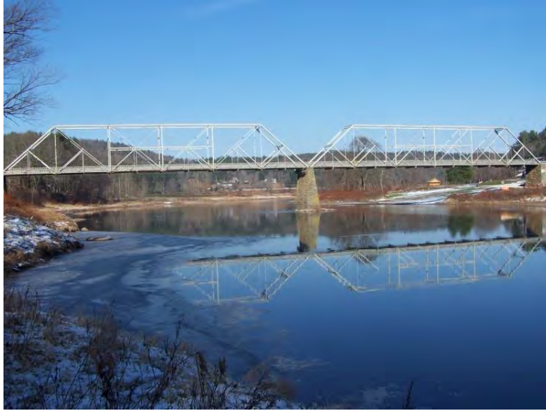
Photo 1 - Skinnners Falls Bridge: Downstream Elevation (Looking North)
