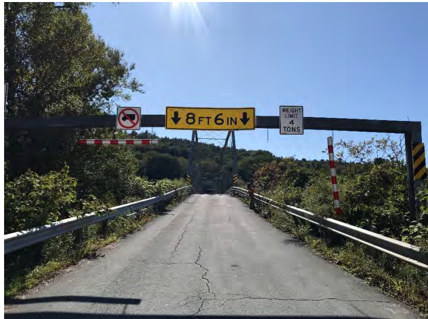
Photo 6 - Skinnners Falls Bridge: Headache Bar at NY Approach
