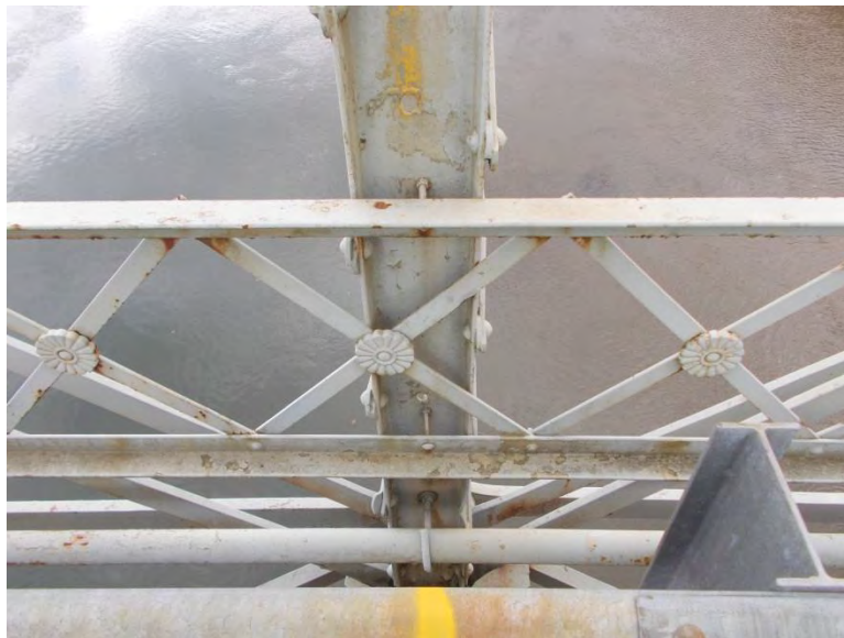
Photo 38 - Skinners Falls Bridge: Railing Bolted to Vertical Truss Member, Span 2
