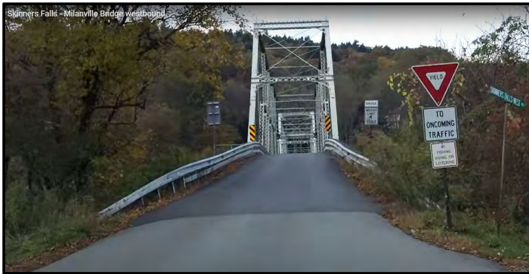
Figure 2: New York Approach geometry with a view west of the approach on the east (New York) side of the bridge.
