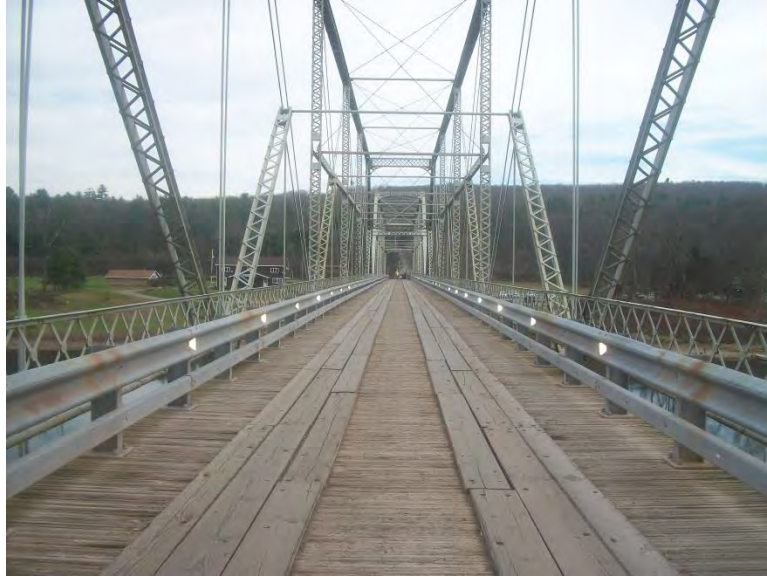
Photo 3 - Skinnners Falls Bridge: Typical Guiderail across Structure Looking Ahead
