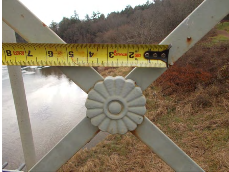
Photo 37 - Skinners Falls Bridge: Close Up View of Rosette (Typical)
