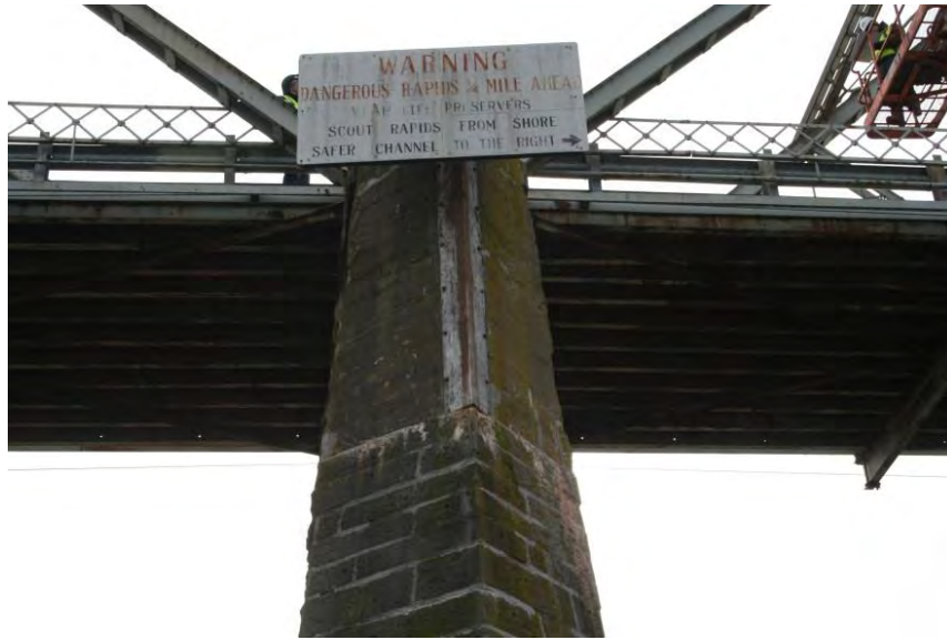
Photo 27 - Skinnners Falls Bridge: Steel Cap at the Top of the Upstream Nose of Pier
