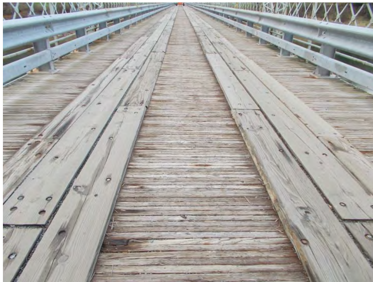
Photo 4 - Skinnners Falls Bridge: Typical Top of Deck and Bridge Rail
