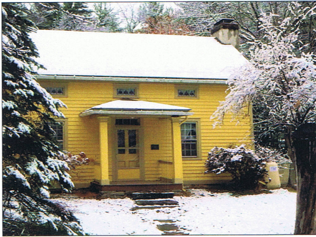
The Nathan Skinner House c. 1815. Nathan partly framed this house seven miles upriver and rafted it to Milanville.
