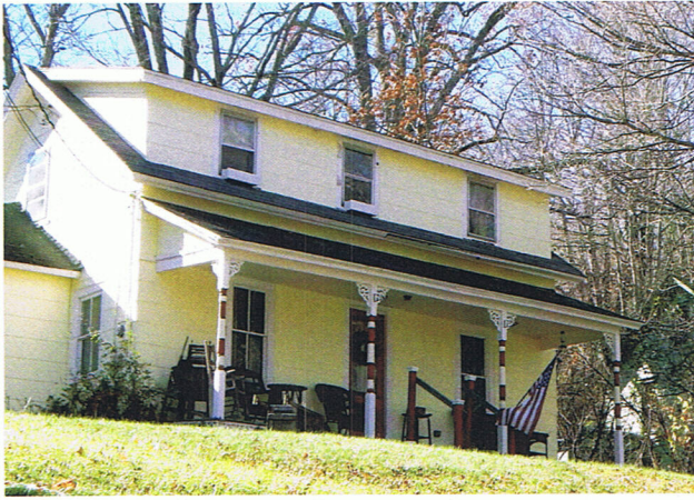
Frank Davis House c. 1900. A side gabled, 1.5 story residence. Just west of the Illman House, on the same knoll.
