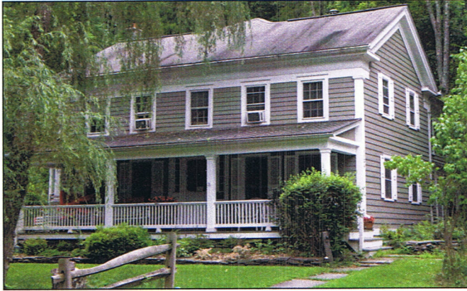
The Eli Beach house c. 1850. Eli Beach owned and operated Milanville's tannery for several decades.
