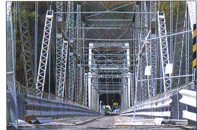
Struts and trusses.
