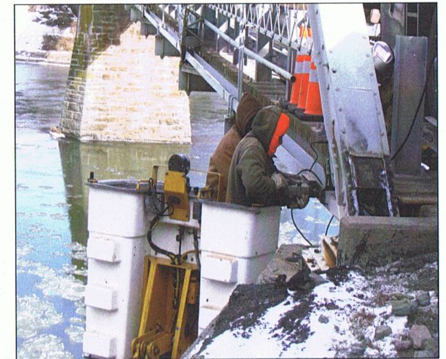
Workmen at the bridge in January 2010. Despite frigid conditions they soon finished the job. Note ice on the Delaware River.
