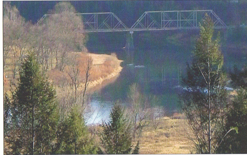
The Milanville Bridge, from a hill 1/2 mile upriver.
