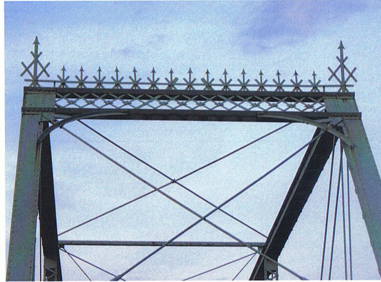
Decorative crests on NY and PA portals.
