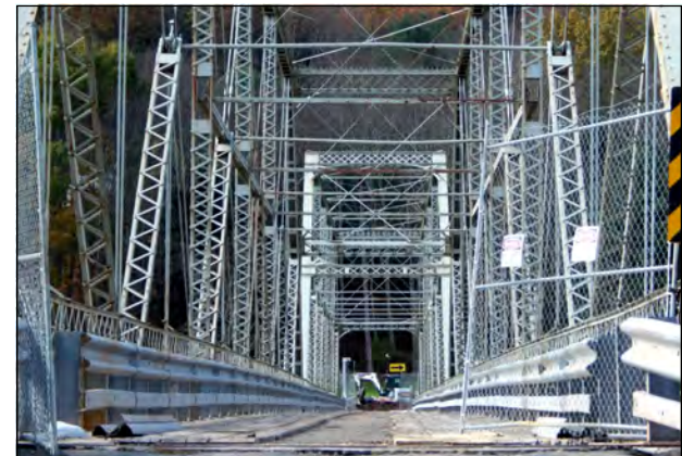
Struts and trusses.
