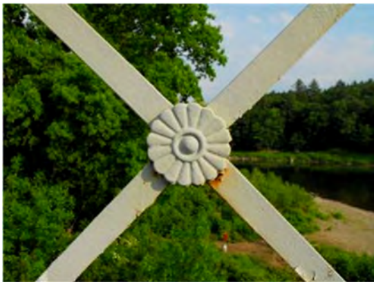
Flower motifs on bridge railings.
