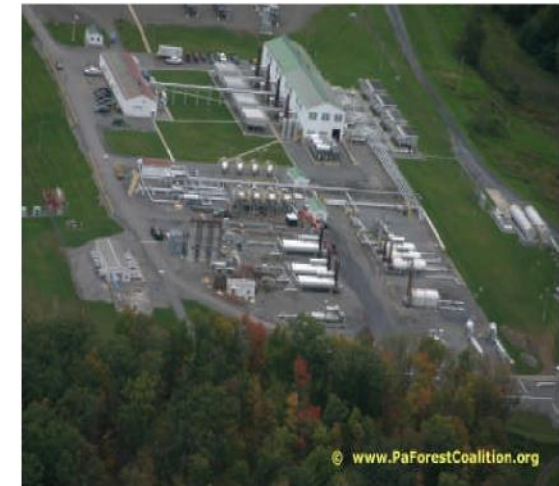
Greenlick Compressor Station Susquehannock State Forest
