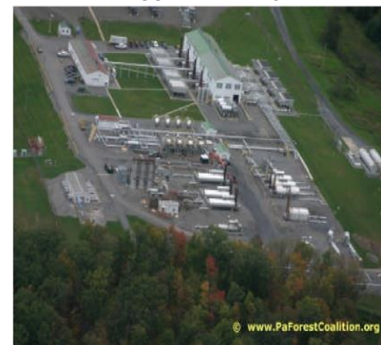
Greenlick Compressor Station Susquehannock State Forest
