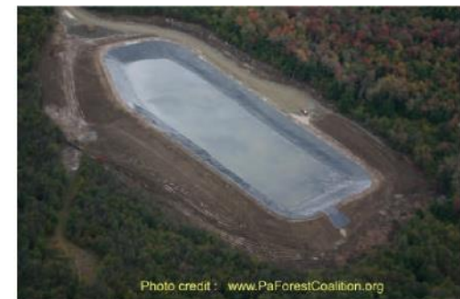
14.5 million gallon fracking reservoir needs to be refilled every third fracking. Note red pickup for scale.
