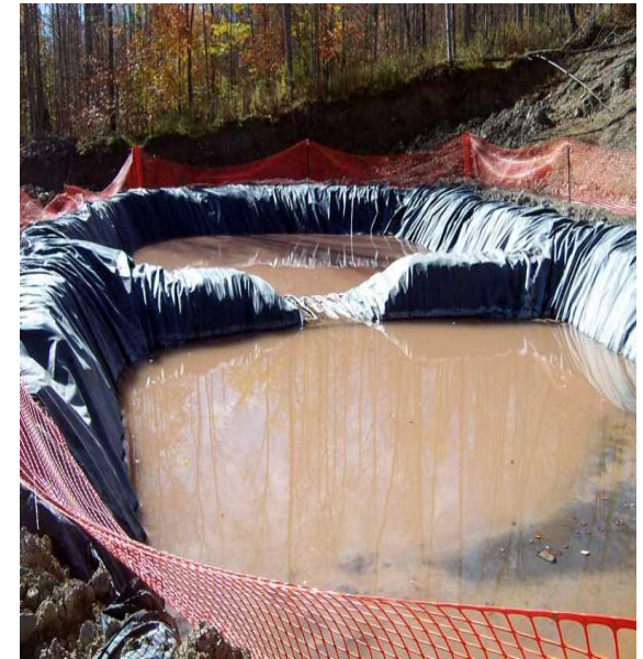
Has your quarry been drinking from drill cutting pits? Open pit on BoosLaw Road, Smyrna, Chenango County
