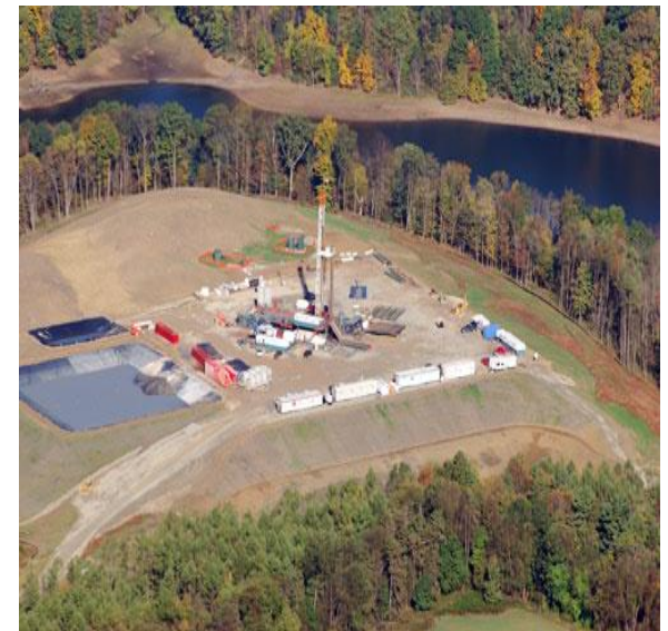
Drill Site next to Beaver Run Water Reservoir, PA
