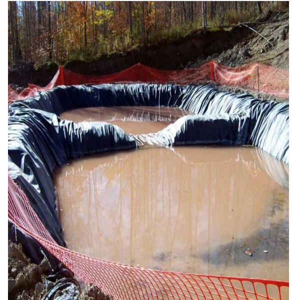
Has your quarry been drinking from drill cutting pits? Open pit on BoosLaw Road, Smyrna, Chenango County
