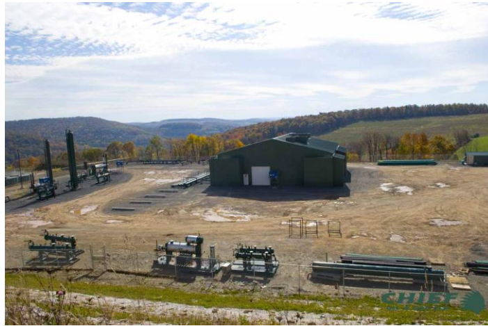
Figure 1. Barto Compressor Station (source: http://www.chiefog.com/cstations.html )
