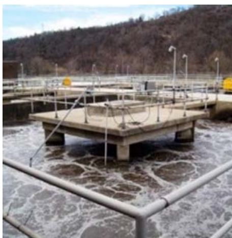
WASTEWATER ONSLAUGHT: The McKeesport Sewage Treatment Plant, one of nine plants on the Monongahela River that has treated wastewater from Marcellus Shale drilling operations. Image: CREDIT: PROPUBLICA/JOAQUIN SAPIEN
