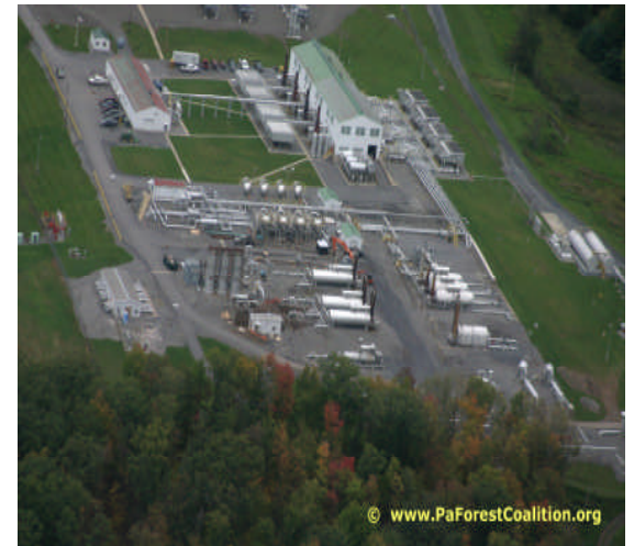
Greenlick Compressor Station Susquehannock State Forest
